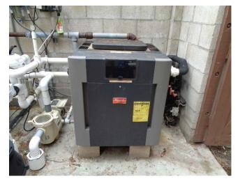
This heater, which has an input capacity of 400K BTU/hr, was replaced during 2011.
