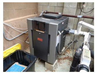
This heater, which has an input capacity of 250K BTU/hr, was replaced between 2015 and 2016.
