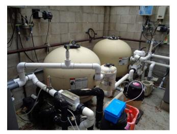
This sand filter, which has a filter surface area of 7.06 sq. ft., was replaced in July 2010.
