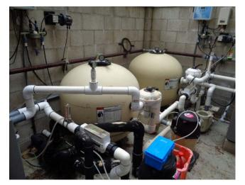
This sand filter, which has a filter surface area of 7.06 sq. ft., was replaced in June 2012.
