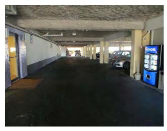
Asphalt was in generally good condition during site visit. Component is for overlay of asphalt areas on 20 year interval. Original 1987 paving was overlaid and restriped in 2006 per client. The actual condition of asphalt areas should be evaluated annually and appropriate repairs performed in a timely manner. Repairs to damaged areas will allow asphalt to achieve the expected useful life.
