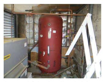
Water heater consists of boiler and storage tank. Both are located in mechanical room on south end of roof. Per client, original water heater life was 26 years. Cost to replace water heater was \$50,000 in 2013.
