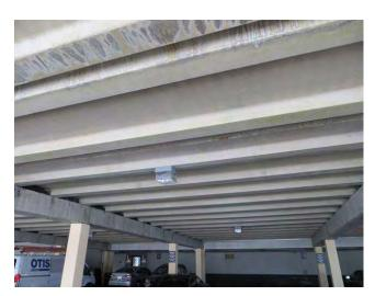
Component covers replacement of original 1987 upper parking level concrete pre-cast slab system. Current experrience with pre-cast slabs is good. Client reports no major issues with structure. One area was repaired over the years. Since it is unlikely that entire structure will have to be replaced, replacement percentage set at 50%. Reduction confirmed by client.
