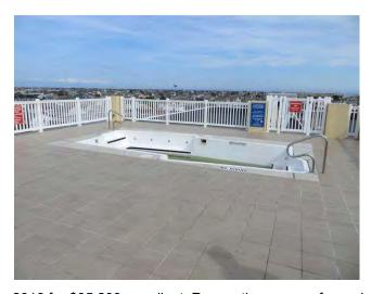
Pool deck area was renovated in 2016 for \$95,200 per client. Renovation was performed due to leaks in roof membrane under pool deck. Renovation included engineering study, new tile and roof membrane in pool area. Approximate 20% of roof covered by pool deck.
