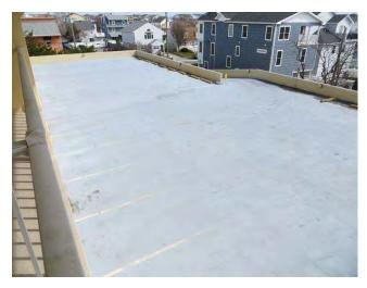
When originally installed in 1987, upper parking level concrete surface was not coated. In 2012, concrete was extensively prepared by grinding and stripping surface. Waterproof Sika sealer was then applied. Component is for replacement of sealer after 15 years. Replacement will not require as much prep work as original installation. A separate component covers inspection and reapplication of sealer on 5 year interval. Replacement interval provided by client.
