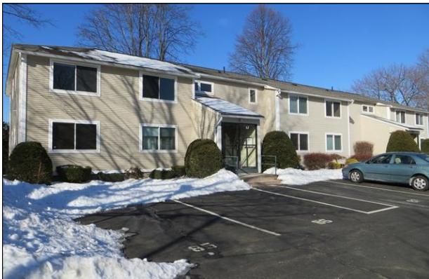
Edgewater Gardens Condominium Association Holyoke, Massachusetts
