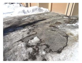
Most asphalt areas can be expected to last approximately 20 to 25 years before it will become necessary for an overlay to be applied or other major rehabilitation to be completed. It will be necessary to adjust manhole and valve covers at the time the overlay is applied or other major rehabilitation is completed.
