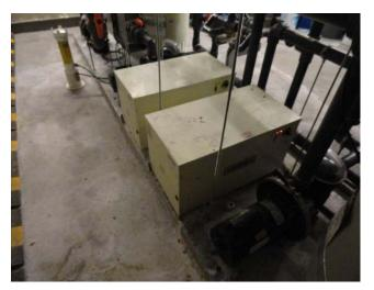
These are Coates electric pool heaters located in the pool equipment room.
