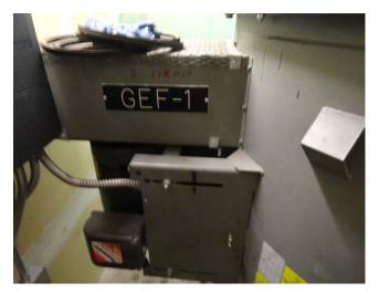
This is GEF-1 power ventilator fan for the lower level. This fan is located in the fan room.
