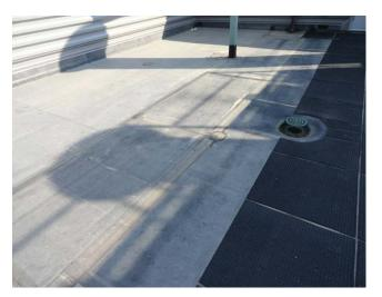
This is the roof on the top of the building. According to the association this is a three ply waterproof membrane roof and installed in 2007.
