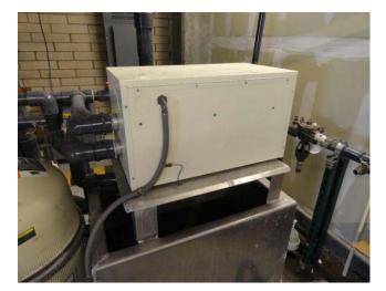
This is a Coates electric spa heater located in the pool equipment room.
