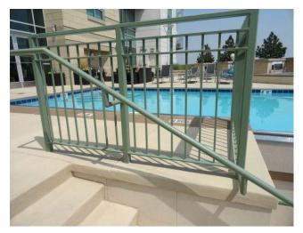
This is standard grade painted tubular steel railing and handrail located in the pool area.
