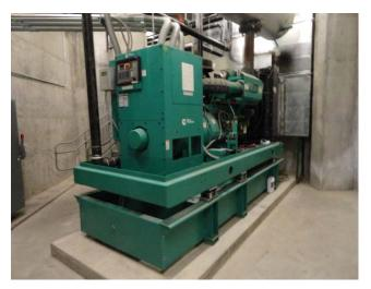
This is a Cummins back up generator located in the generator room. This is a model #DFEK-5768223. This is for a major refurbishment of the generator to include engine and alternator.
