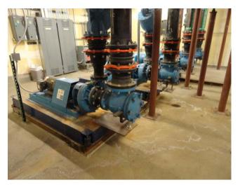
These are Baldor 15hp pumps located in the roof top equipment room that service the cooling towers.
