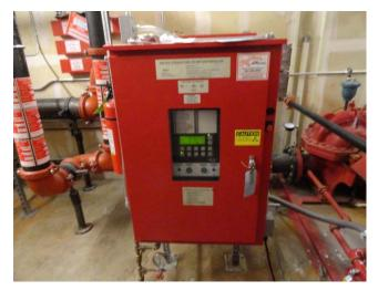
This is a Metron Inc. Model FD4-J fire control panel located in the fire room.
