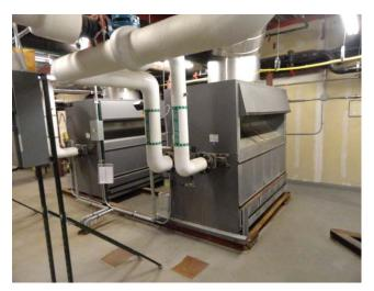
B-1 & B-2 are the boilers that service the condensing loop. Boilers DWH-1 & DWH-2 service the domestic hot water. These are LAARS natural gas boilers that have a BTU/input between 3,050,000 & 3,500,000 per hour.
