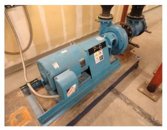
These are Baldor 30hp pumps located in the roof top equipment room that service the closed loop water.
