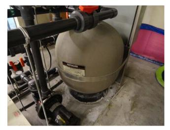
This is a Hayward commercial high rate pool sand filter located in the pool equipment room.
