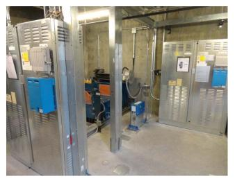
These are Otis traction style elevators located in the roof top equipment room.
