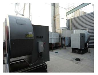
These are identified as SEF-1, HPF-3 & SPF-2B located on the roof. Two service the elevator shafts and one services the roof top equipment room. Each fan has a 20hp motor.
