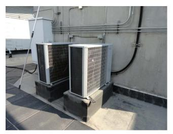
These are identified as U-21 & U22 HVAC units that service the elevator rooms on the roof top.
