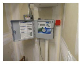
This is a Hunter ICC 28 zone controller located in the fire equipment room.
