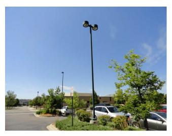
These are aluminum, box style, 400 watt vapor light fixtures with baked enamel finish.
