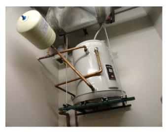
This is a Bradford/White 40g natural gas hot water heater located in the janitors closet.
