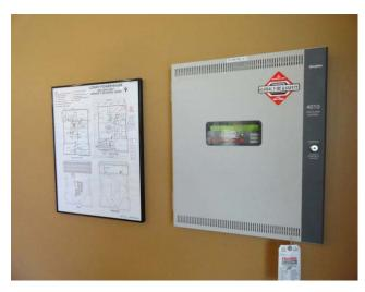
This is a Simplex 4010 fire alarm control panel located on the first floor of the building.
