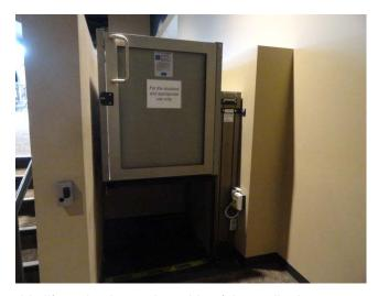
This is a Garaventa two stop portable lift station located outside of the auditorium.
