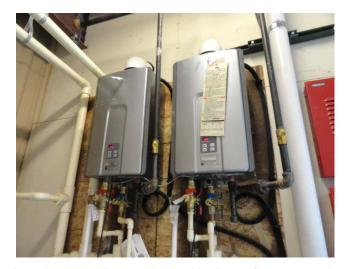
These are Rinnai tankless natural gas hot water heaters located in the roof access equipment room.
